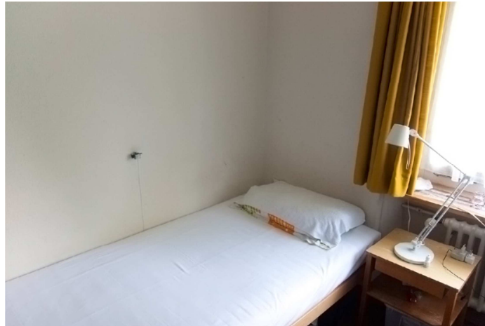
Figure 5-21 Passive sensor node installed next to the bed
