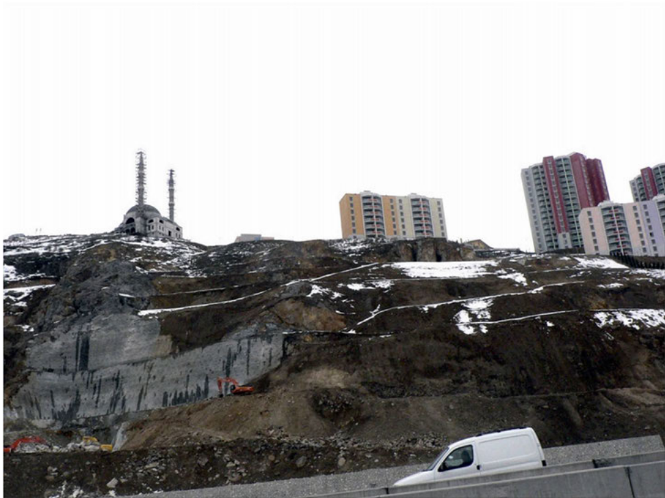
Figure 3: Tearing down the gecekondu for urban transformation project (Mendilcioğlu, 2011).
