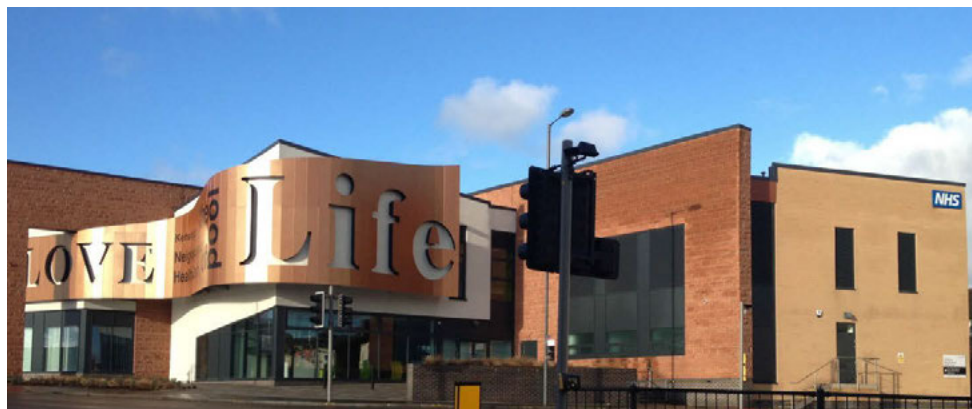
Figure 3: Kensington Neighbourhood Health Centre (Source: Maliene, 2014)
