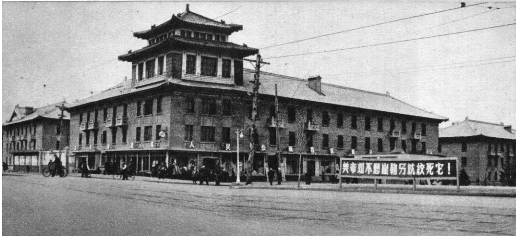
Figure 2-18 Housing at the First Automobile Works, Changchun, 1953-1956
