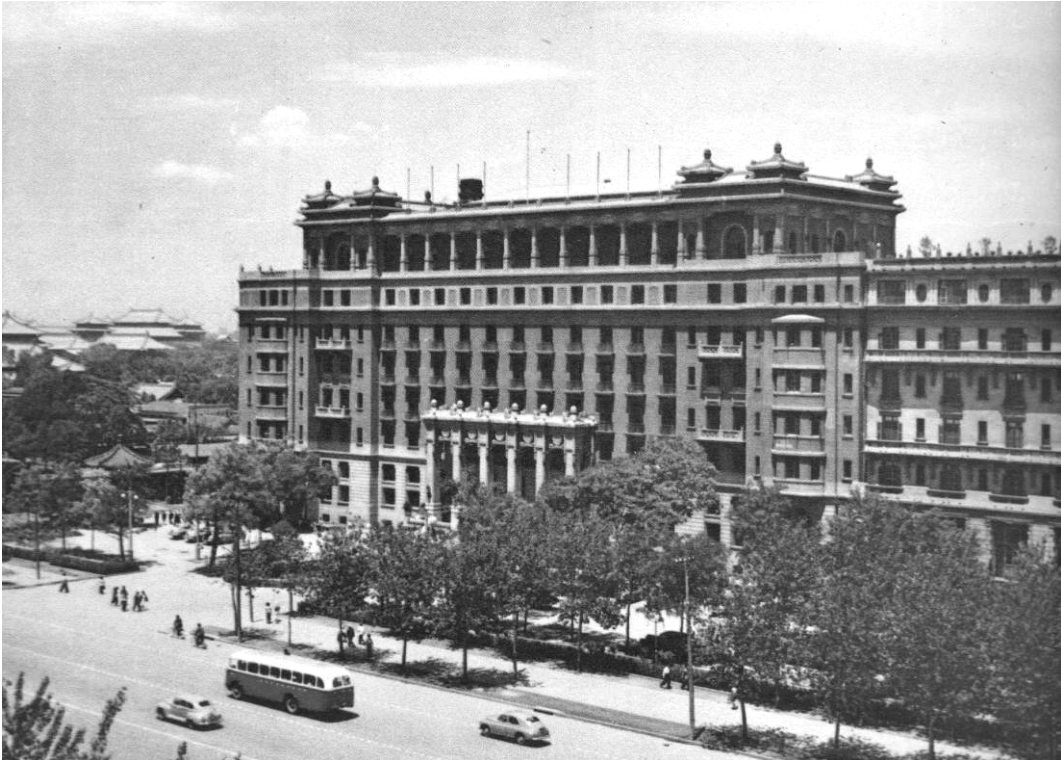
Figure 2-22 West Building of Beijing Hotel, Beijing, 1953-1954, Dai Nianci
