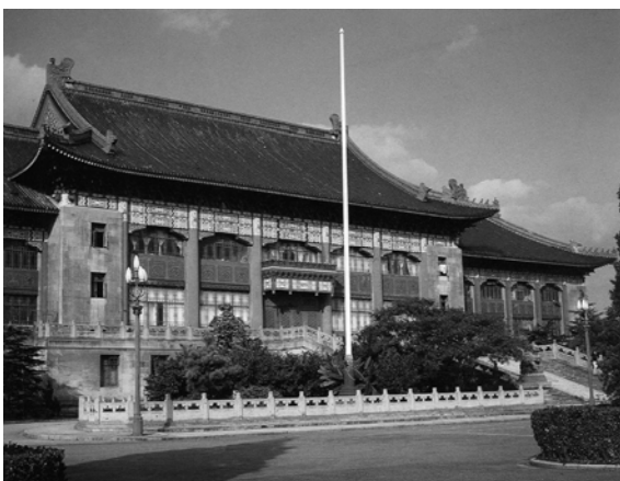
Figure 1-51 Municipal Hall, Shanghai, 1931-33, Dong Dayou
