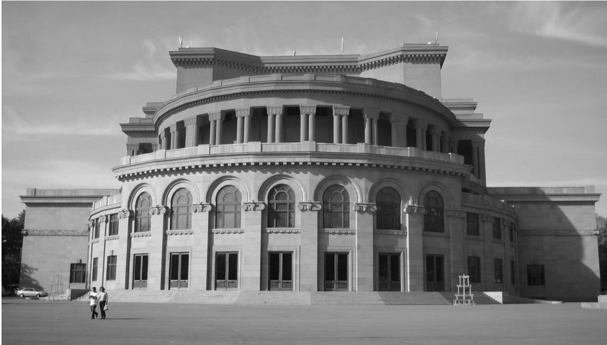
Figure 2-12 Opera House, Yerevan, 1929-1936, A. Tamanian
