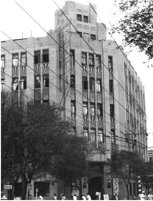
Figure 1-85 Sin-Hua Trust & Savings Bank, Tianjin, 1934-35, Shen Liyuan
