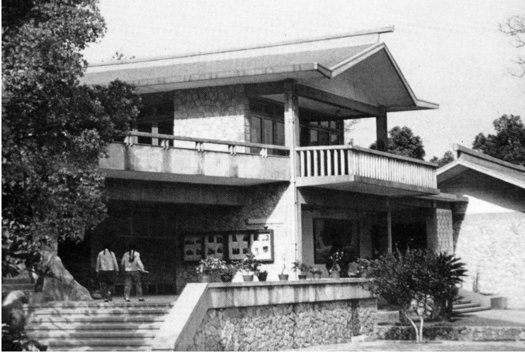
Figure 3-39 Rest House at Ludiyan Park, Guilin, 1963, East China Design Institute for Industrial Architecture, Shanghai Design Institute for Civil Architecture, and Tongji University
