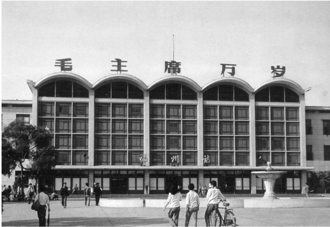
Figure 3-22 Fuzhou Railway Station, Fuzhou, 1959, Huang Xiaoxiu
