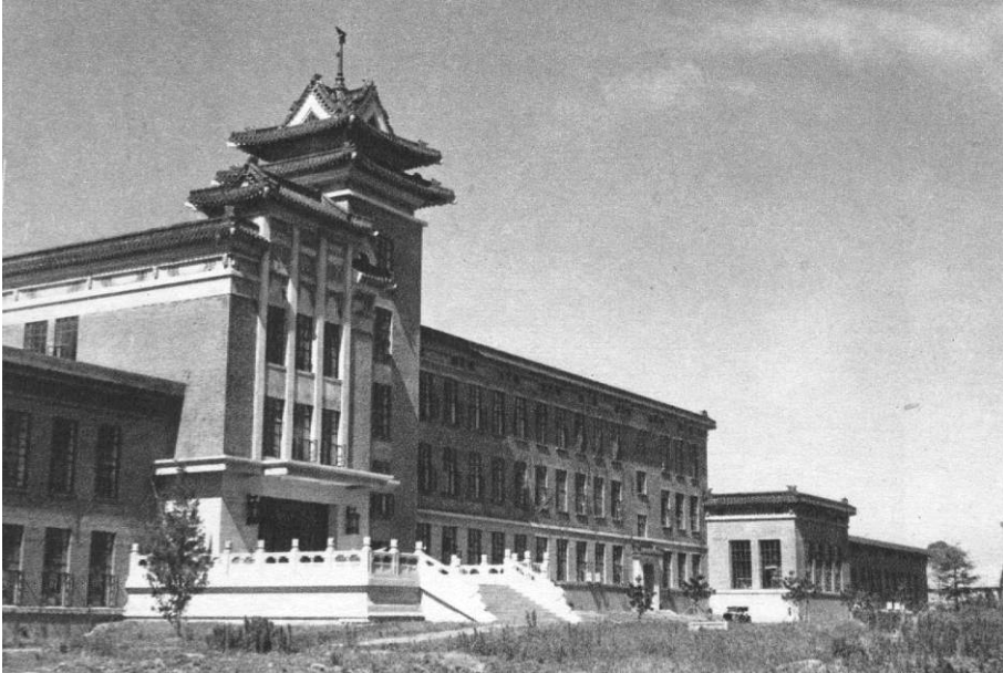
Figure 2-25 Classroom Building at East China Aeronautical College, Nanjing, 1953, Yang Tingbao
