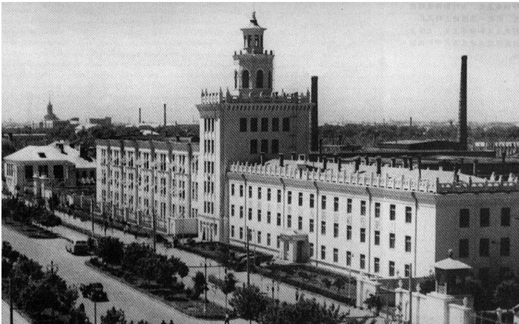
Figure 2-17 Office Building of Harbin Measuring and Cutting Tool Works, Harbin, 1954
