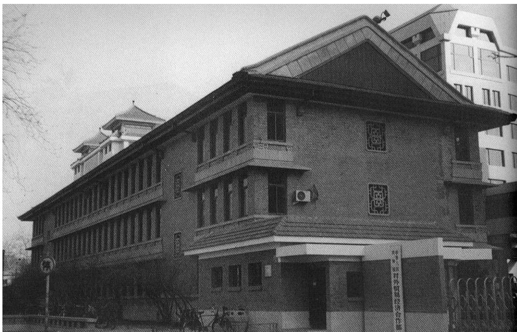
Figure 3-27 An Office Building of the Ministry of Foreign Trade, Beijing, 1952-1954, Xu Zhong
