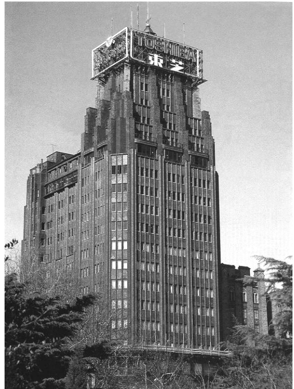
Figure 1-68 Joint Saving Society Building, Shanghai, 1931-1934, L. E. Hudec
